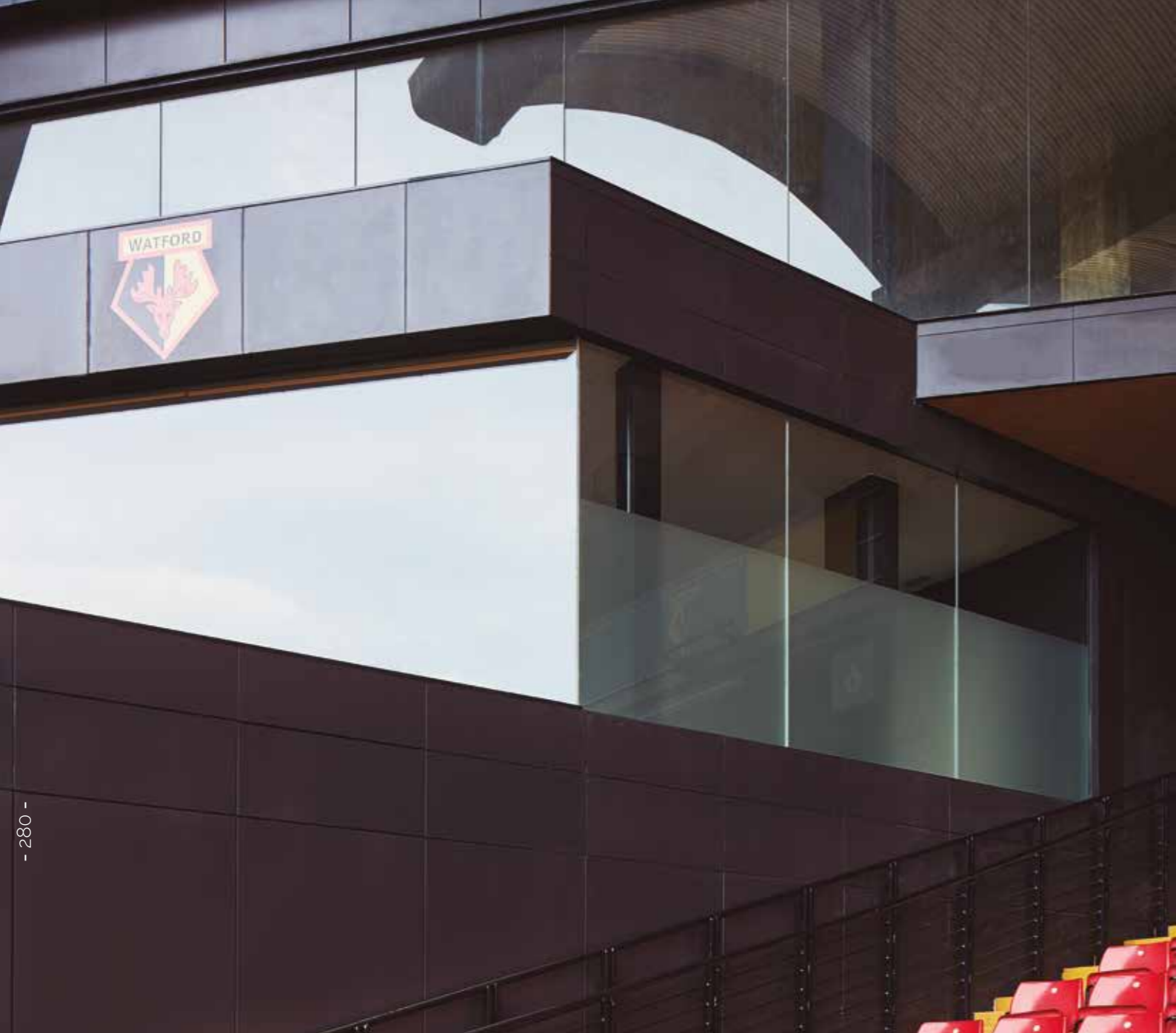
Project: Vicarage Road Stadium (Watford FC) . Hertfordshire (Reino Unido)
